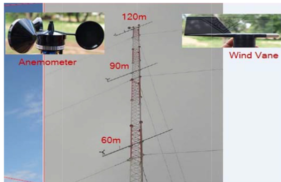
Figure 2 Wind mast and all equipments
